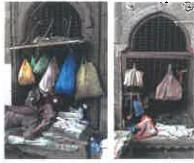
MISUSE OF GATEWAYS AND ARCHED WINDOWS.
