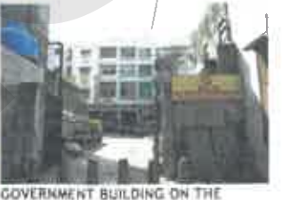
GOVERNMENT BUILDING ON THE STREET ADJOINING PREMABHAI HALL.
