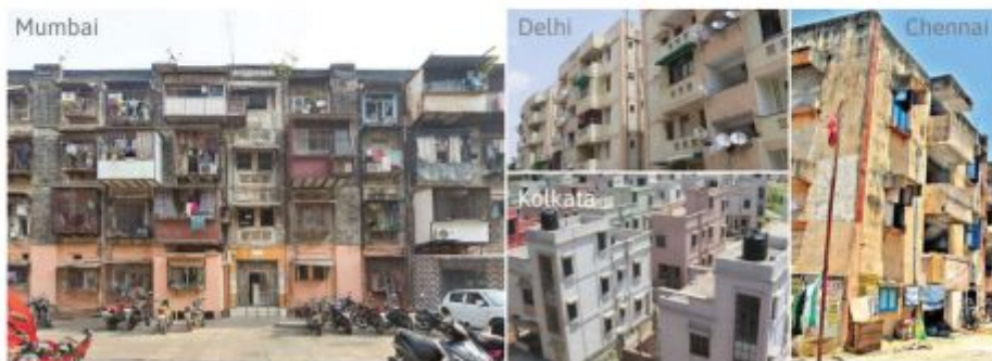
Figure3: Images showing residential buildings of different cities in India.
